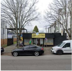
12 | 5435 California Ave SW | Commercial (Form and Material)
