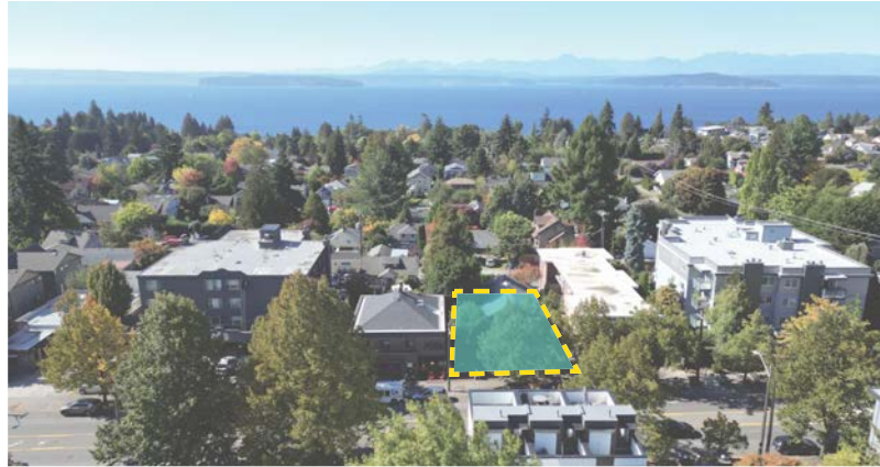
2 ~ AERIAL LOOKING WEST
