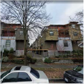
8 | 5920 California Ave SW | Multi Family Residential (Central Circulation)
