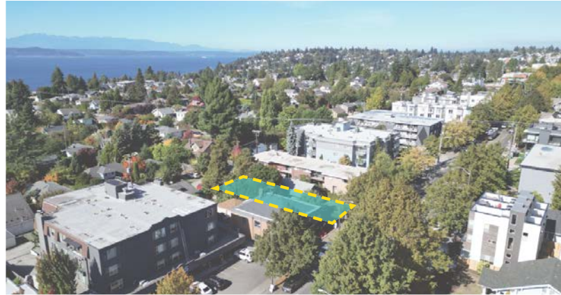
3 ~ AERIAL LOOKING NORTHWEST
