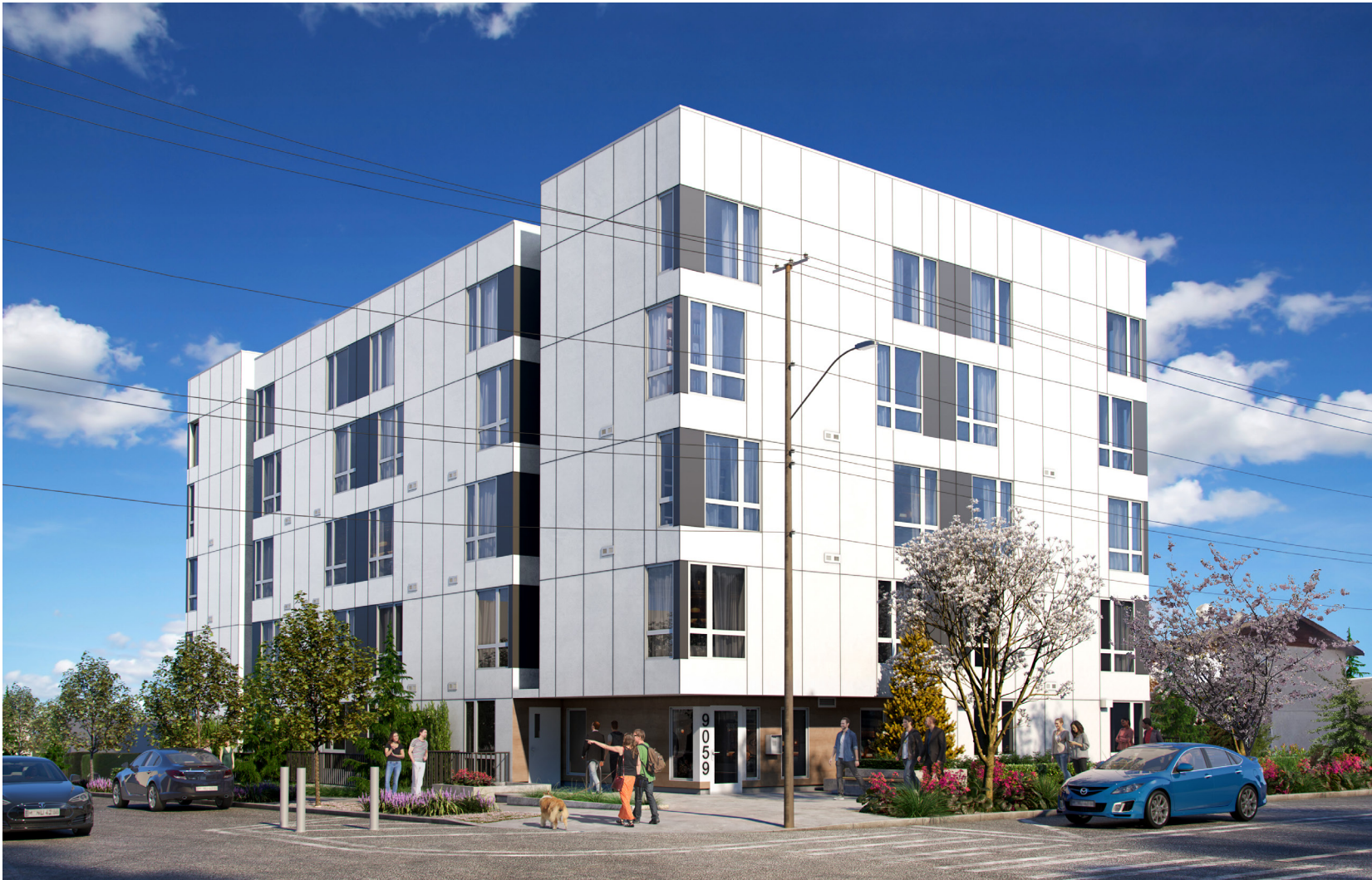
9057-9059 16th Ave SW 3039754-LU 1. Fiber cement panel, BM Chantilly Lace, smooth finish 2. Fiber cement panel, BM Jet Black, smooth finish 3. Vinyl window, white 4. C Clear cedar privacy fence, clear finish 5. VG Clear cedar siding, horizontal, Cabot Semi-Transparent Stain Ultra White
