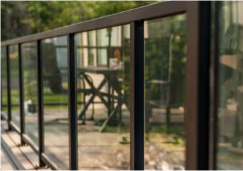
GLAZED GUARDRAIL W/ DARK BRONZE ALUMINUM FRAME
