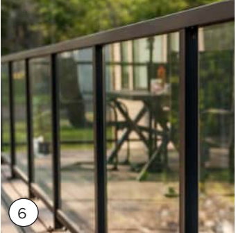
AREA A, C 42\" Glazed Guardrail with Dark Bronze, Aluminum Frame
