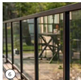
6 42" Glazed Guardrail with Dark Bronze, Aluminum Frame
