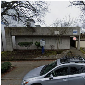
11 | 5429 California Ave SW | Commercial (Form and Material)
