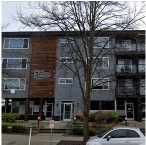
2 | 5600 California Ave SW | Multi Family Residential (Material)
