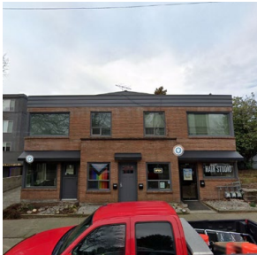
14 | 5619 California Ave SW | Commercial (Material)
