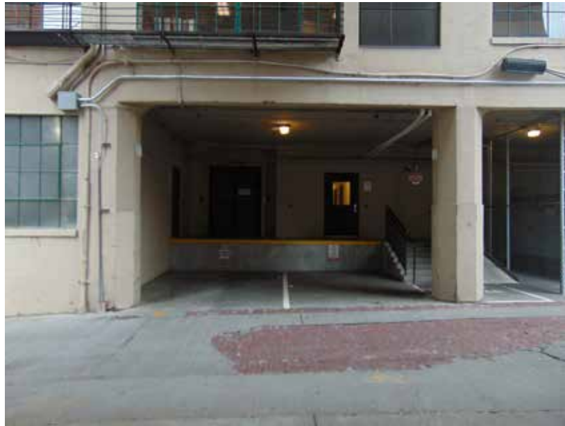
VIEW EXITING PORTE COCHERE
