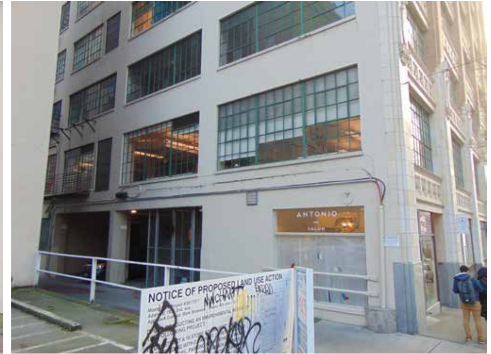
TERMINAL SALES BUILDING - RETAIL @ CORNER
