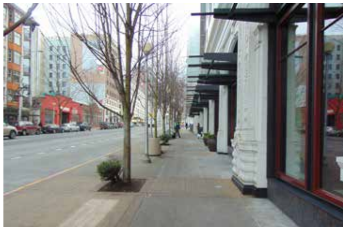
B1 Respond to the neighborhood context. The building responds to the neighborhood with a stone-clad base, matching the materiality of the many landmark buildings in the area. It also provides a similar rhythm of retail bays along second avenue.
