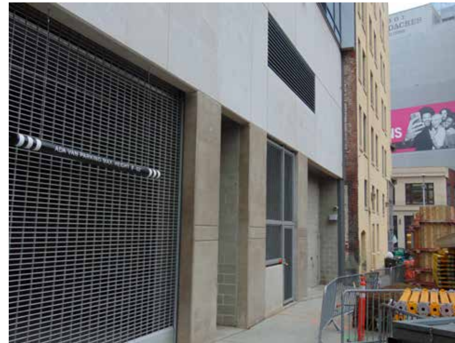
THE VIKTORIA - GARAGE, EGRESS, UTILITY METER
