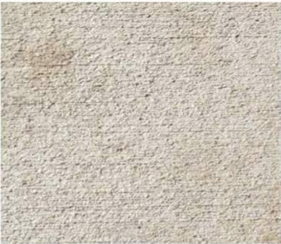
CONCRETE TOPPING SLAB AT PET AREA
