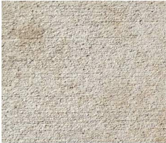
CONCRETE TOPPING SLAB AT PET AREA
