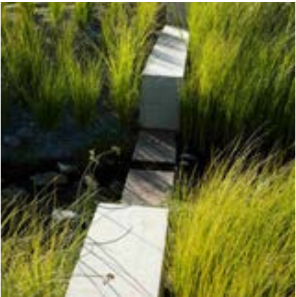
Stepped bioretention planters
