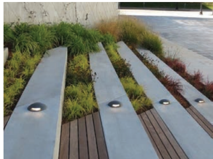
② Embedded Lights - Stair Treads
