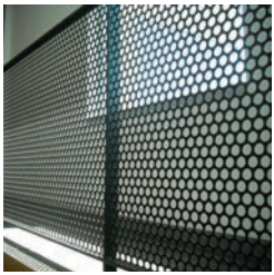
⑧ Perforated Guardrail
