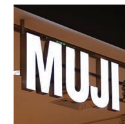
④ Grocery Facelit Aluminum Letters Pin-Mounted to Canopy
