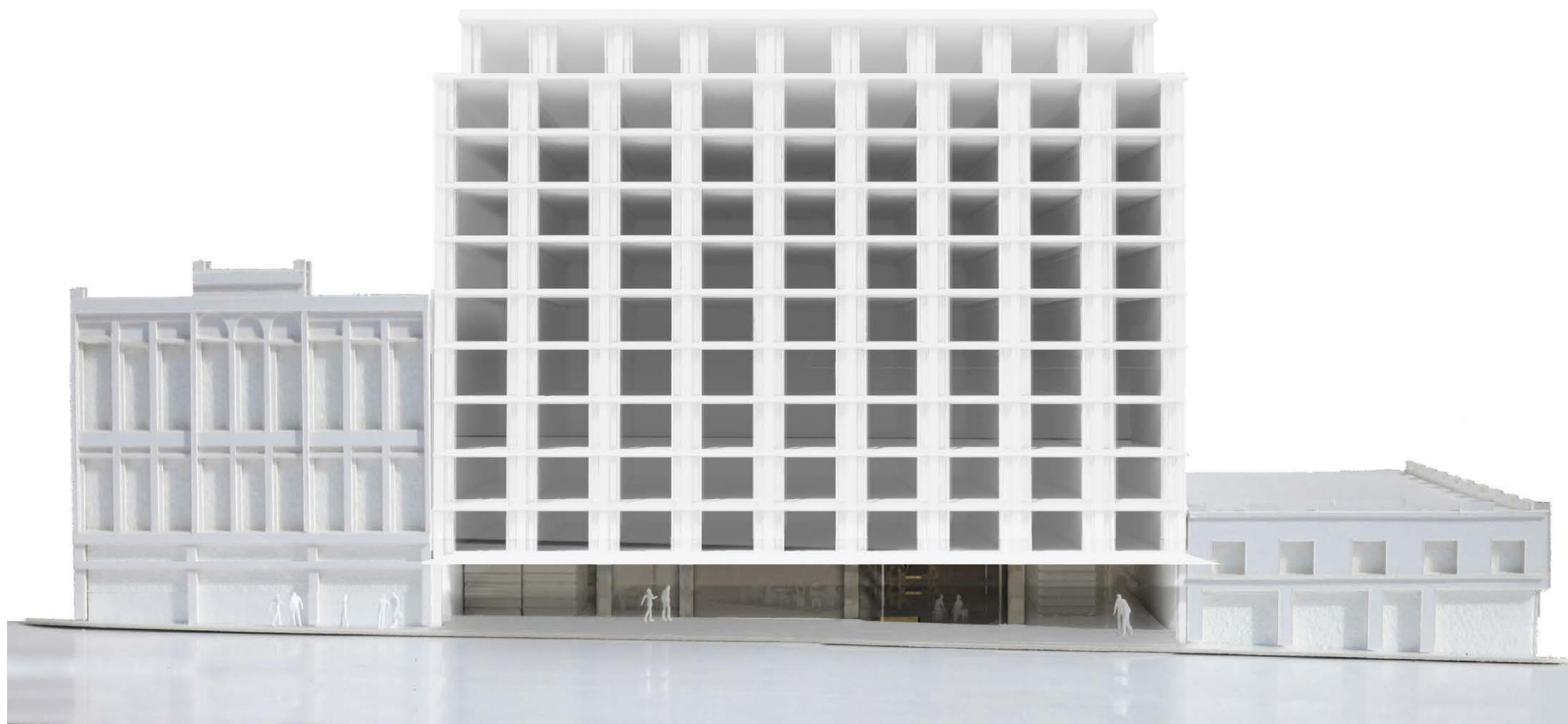
The building's three components, the Forum (ground floor levels), the Apartment House (residential levels) and the Communal Roof (rooftop level) are all clearly legible on the 1st Avenue facade.
