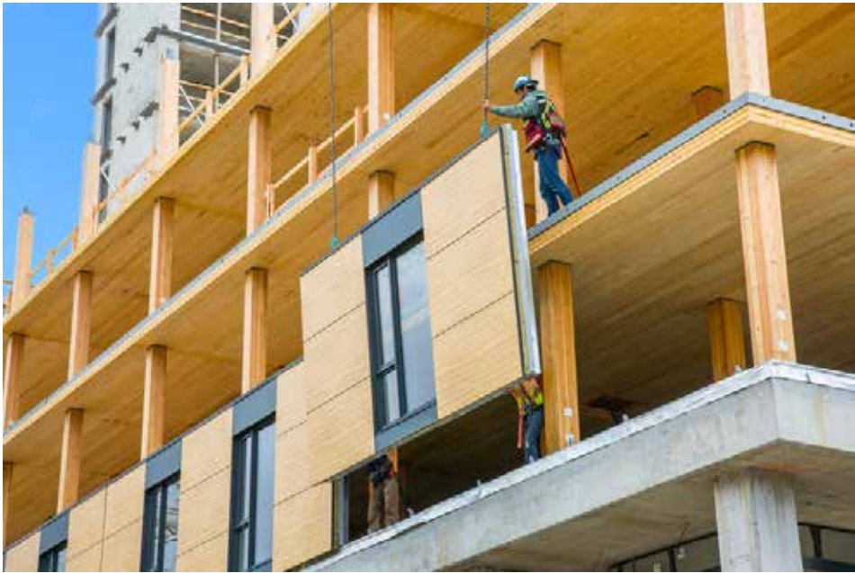
Brock Commons precedent: easy assembly/disassembly of mass timber structure
