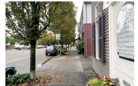
6. Greenwood Ave East - sidewalk condition
