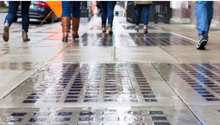
Glass blocks in paving will allow daylight in the parking garage.
