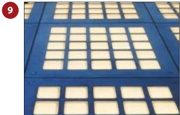
Glass Blocks - Glass blocks integrated into paving provide wayfinding within plaza.
