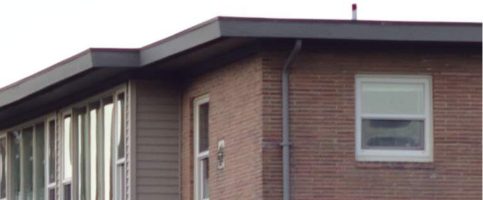
In a typical project, stormwater is directed from roof to gutters and downspouts then to a storm drain or a combined sewer/storm drain.
