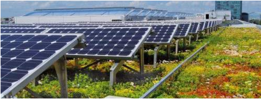
Living Building Pilot options include rooftop solar panels to generate power and reduce energy consumption, and a green roof to treat rainwater underneath.
