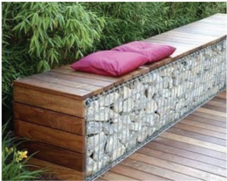
SEAT OVER GABION WALL
