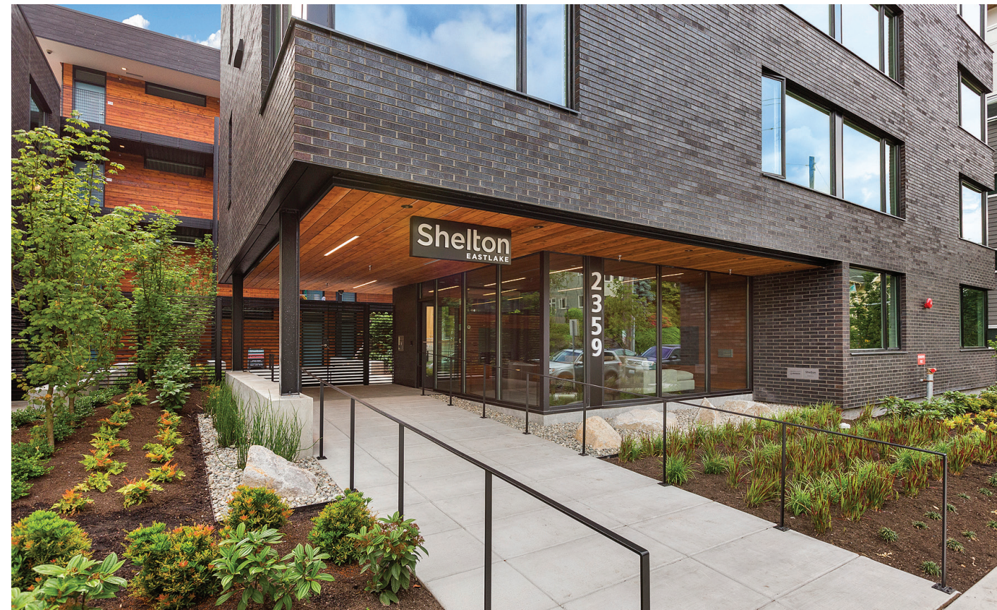
Shelton Apartments Seattle, WA
