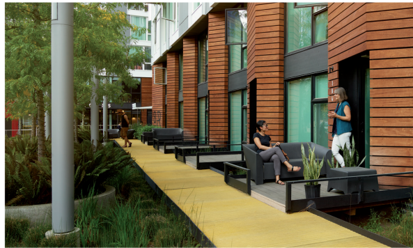
UNIT TERRACES ADJACENT TO BIORETENTION
