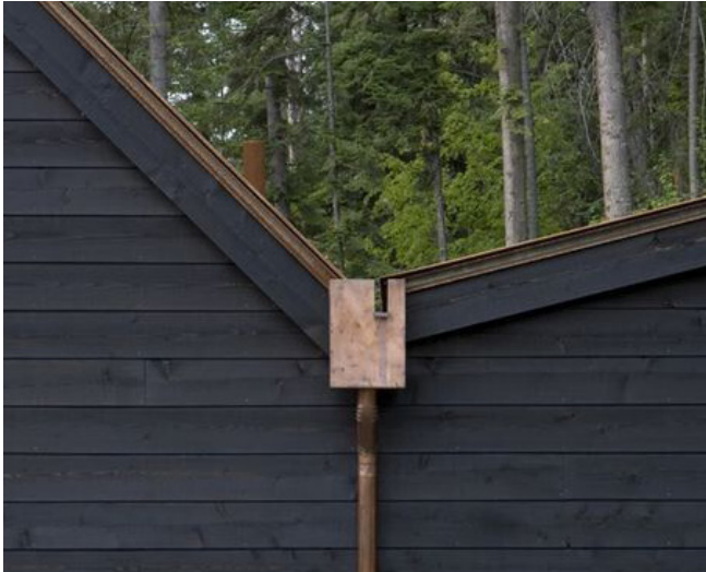
EXPOSED SCUPPER & DOWNSPOUTS RESIDENTIAL SCALE DETAILS
