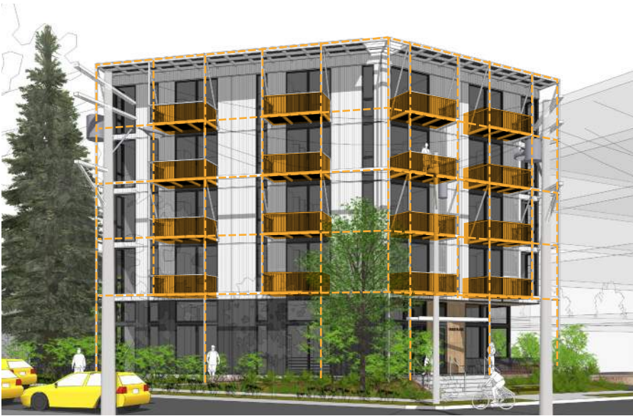
External Framework and Balconies Maintained on the facade.
