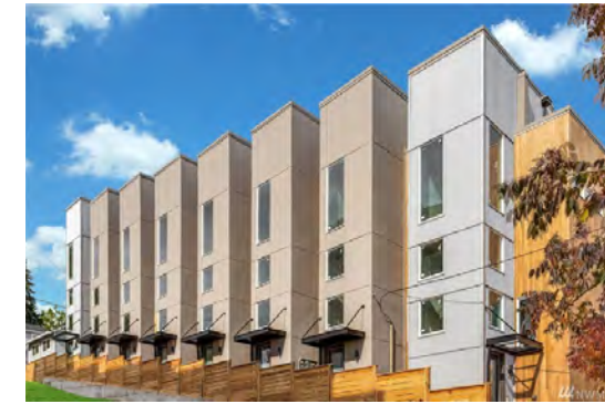
2- SW AVALON WAY TOWNHOMES 3078 SW AVALON WAY | TOWNHOMES 8 Townhouses, units entries face a shared walkway to the south. All units have a patio space at the ground level on the North side.
