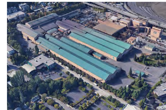
8- NUCOR STEEL 2424 SW ANDOVER ST | SOCIAL SERVICES Steel plant dating back from 1904. Produces steel products for several industries.
