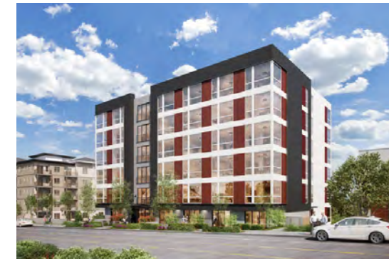
5- 3039 SW AVALON WAY 3039 SW AVALON WAY | APARTMENTS The proposed building is a 7-story apartment building with parking for 19 vehicles below grade, which will be accessed via a ramp off Avalon Way.
