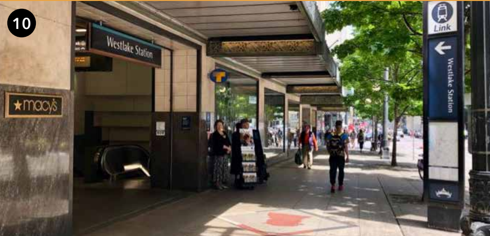
WESTLAKE LIGHT RAIL STATION
