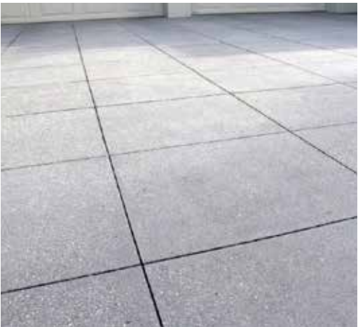
SANDBLASTED AND SAW CUT CONCRETE PAVING
