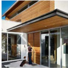
Canopy - Steel Channel/Wood Soffit
