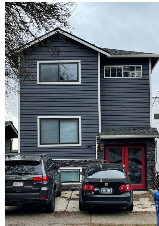
10 SINGLE FAMILY HOME 1215 N 43rd Street
