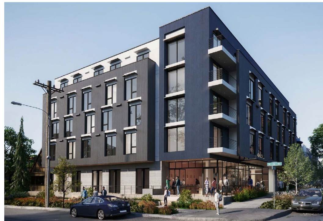
③ WALLINGFORD MIXED-USE (UNDER CONSTRUCTION) 4205 Stone Way N, Seattle, WA 98103
