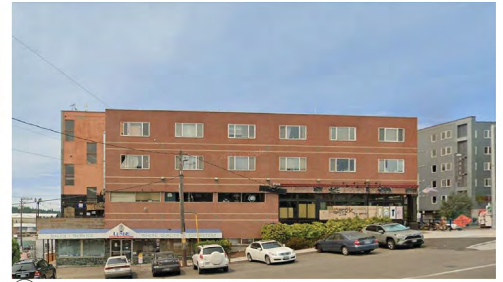
④ LOOKING WEST ON 24TH AVE. NW
