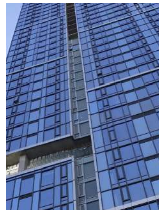
Possible to use spandrel glass to give simple exterior forms articulated by recessed gaskets at intersections and plane changes
