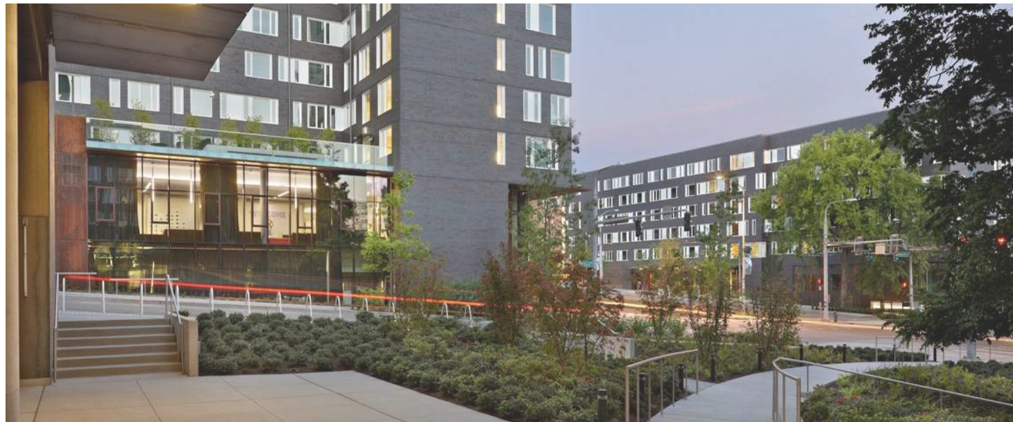
UW West Campus Residence Halls
