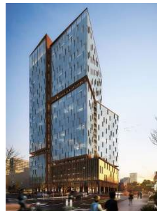
Possible to use spandrel glass to give simple exterior forms articulated by recessed gaskets at intersections and plane changes
