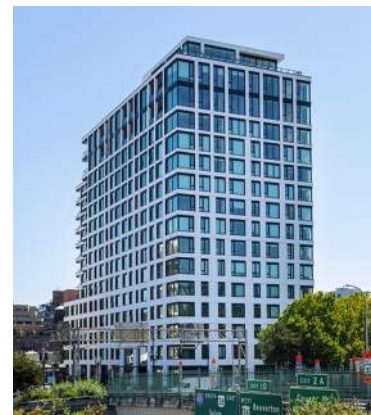
Frame and spandrel/vision glass grid infill as more classic modern - light and forward looking
