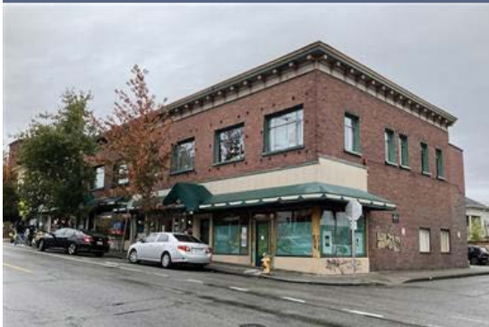
7 Northfield Block 4250 Fremont Ave N
