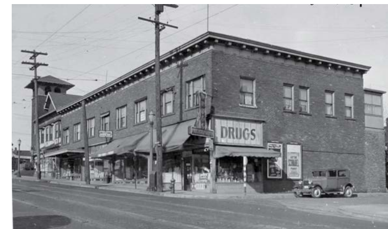
7 Northfield Block 4250 Fremont Ave N year built: 1909
