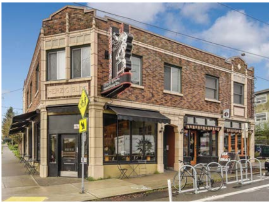
6 Herzing Building 4301 Fremont Ave N
