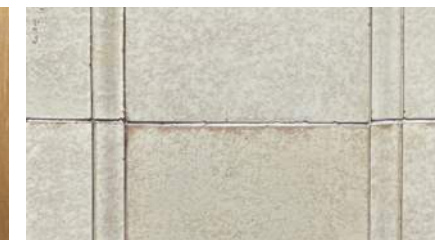
3. Existing Terra Cotta (Cream)
