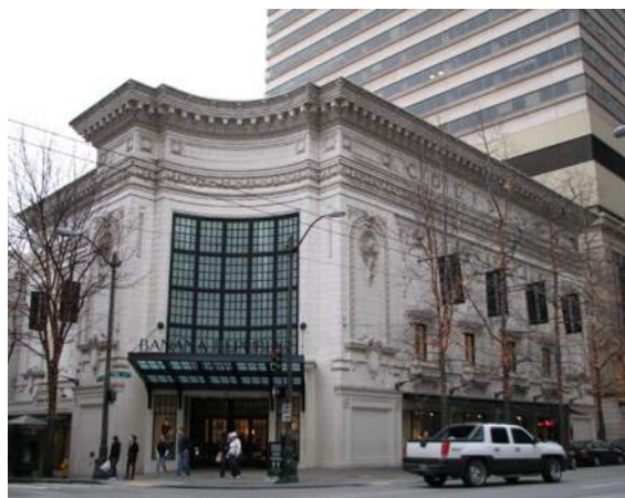
7. Coliseum Theater Building
