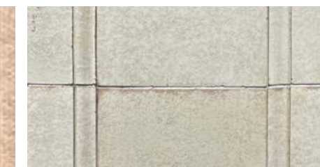
7. Existing Terra Cotta (Cream)
