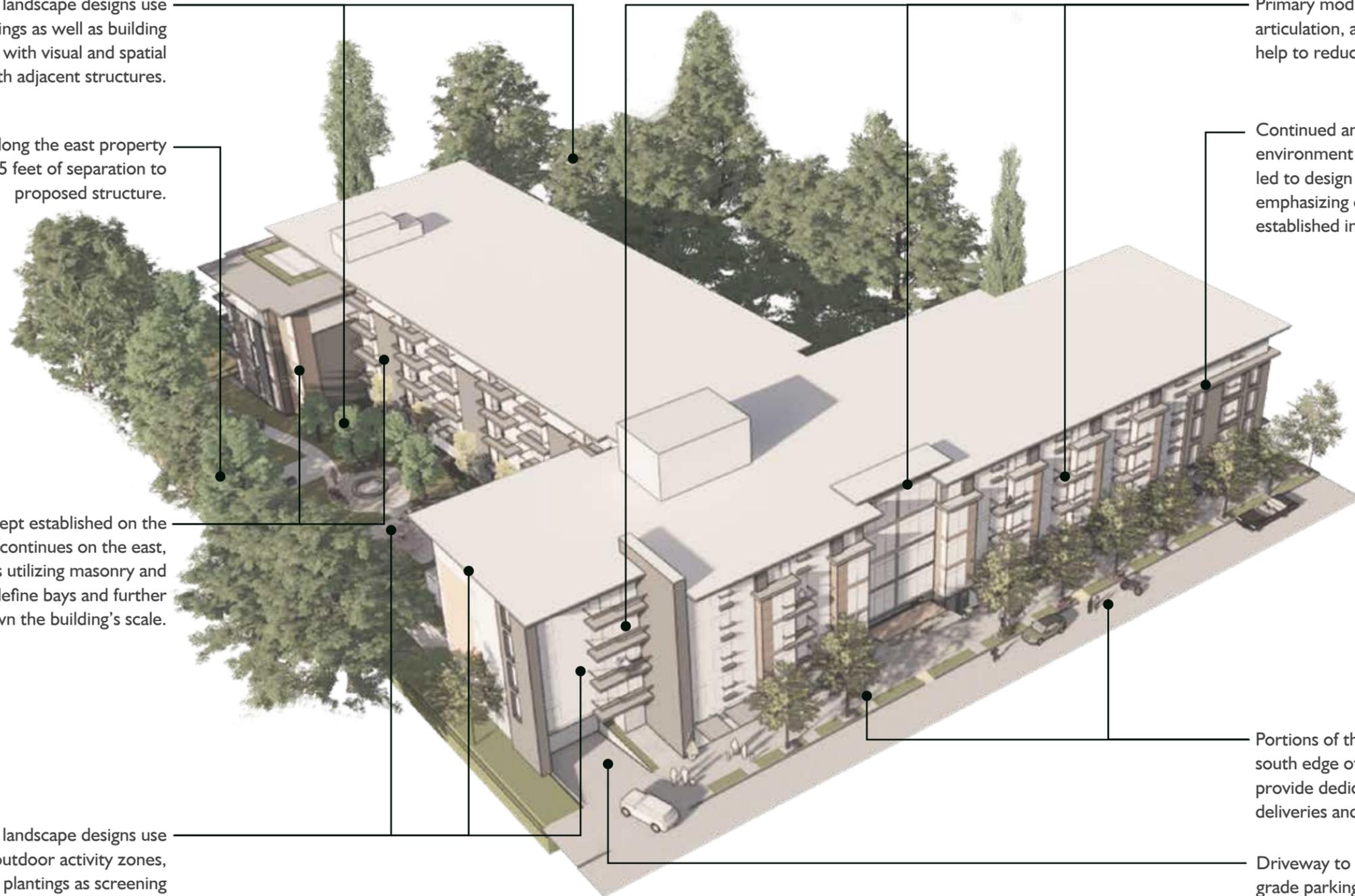
Primary modulation and secondary materials and articulation, along with balconies and roof eaves, help to reduce the overall mass of the north facade.
