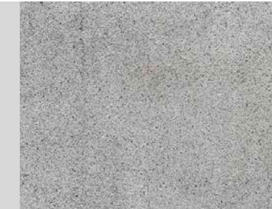
Standard CIP Concrete with broadcast silica and light topcast finish
