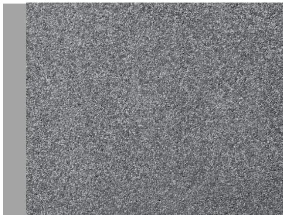
Integral color CIP Concrete with broadcast silica and heavy topcast finish
