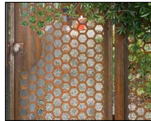
DECORATIVE FENCE LOCAL ARTIST, BOD: PERFORATED CORTEN FENCE & GATE
