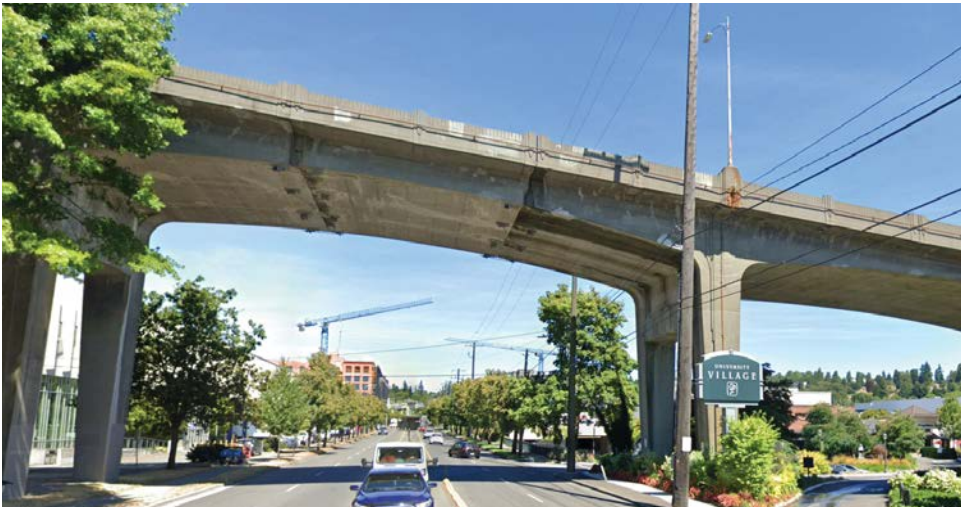
4 45th Street Viaduct.
