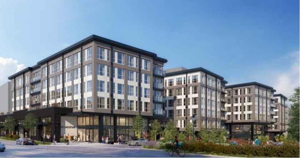
16 4906 25th Ave NE | Strata (under construction)
