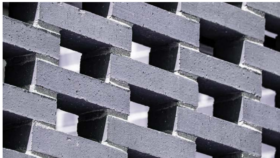
EXAMPLE OF BRICK LATTICE WALL
