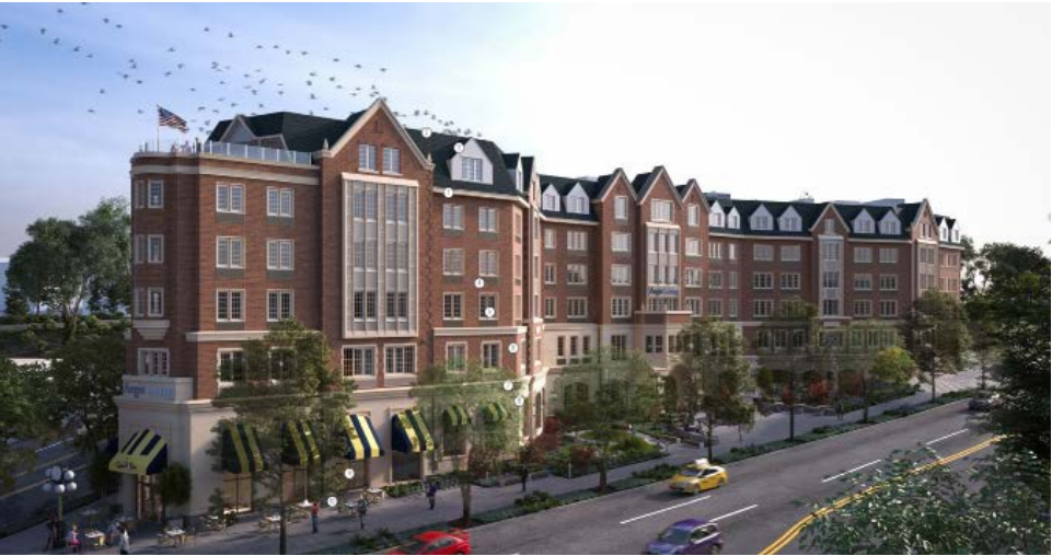
15 3200 NE 45th Street | Aegis Living Laurelhurst (under construction)
