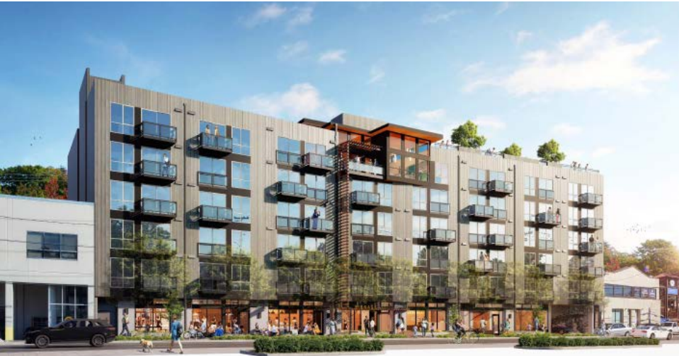
13 4600 Union Bay Place | Spur (under construction)
