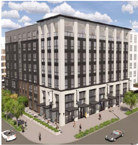
17 4715 25th Ave NE | Arista (under construction)
