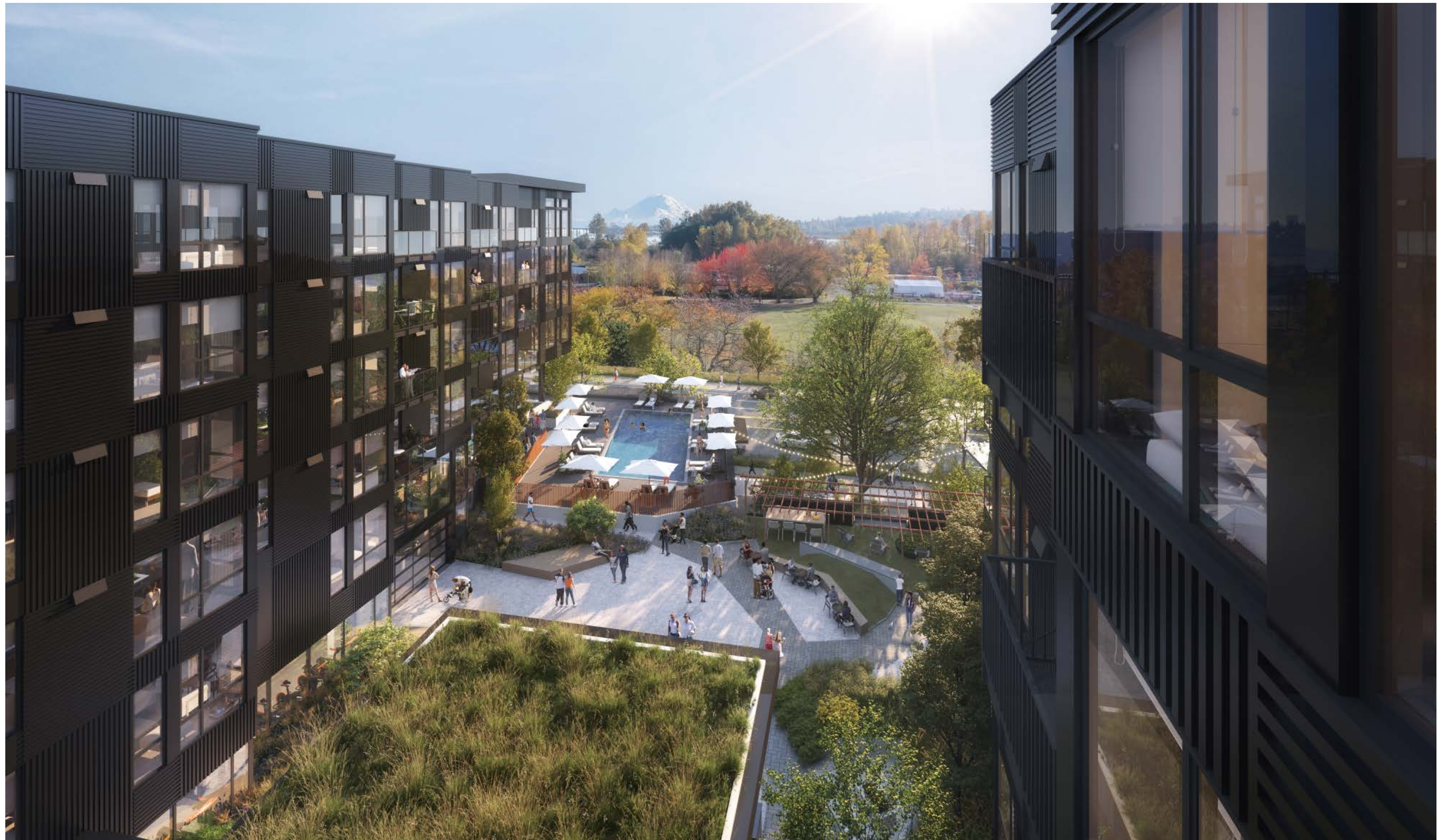
UPPER COURTYARD LOOKING SOUTH
