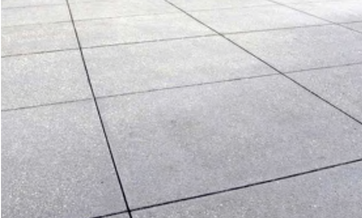
Saw-Cut Concrete
