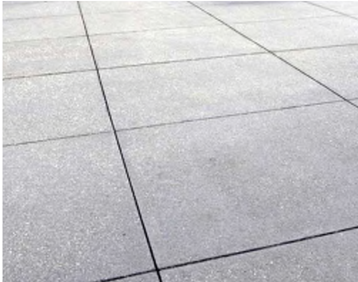
Saw-Cut Concrete
