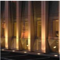
3 Integrated Uplight at Columns Recessed uplighting at columns, creating beam of light at metal panel to signify facade rhythm
