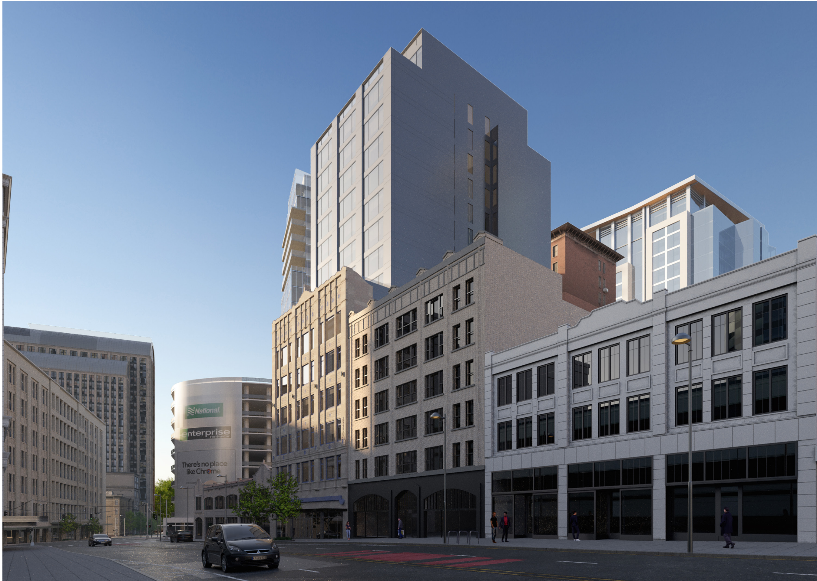
← View from 3rd Ave. and Virginia St.
