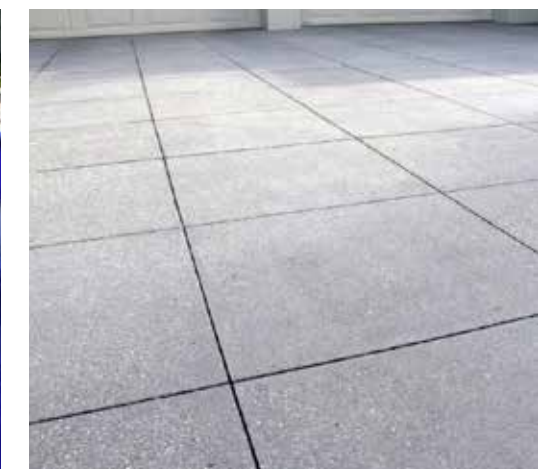
SANDBLASTED AND SAW CUT CONCRETE PAVING
